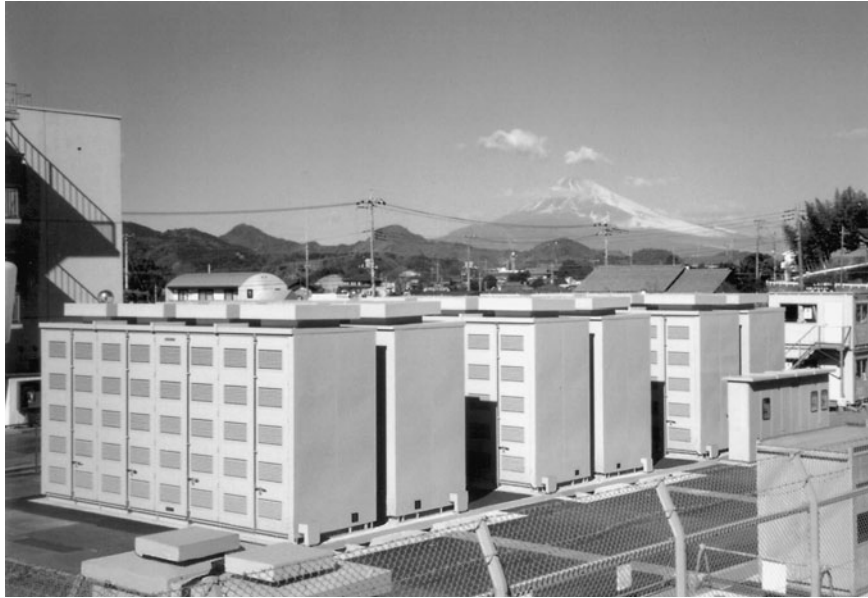
FIGURE 40.16 A photograph a 6 MW/ 48 MWh NGK sodium/sulfur battery system that is operating in a load-leveling mode at Ohito, Japan. This battery is one of the two largest sodium/sulfur batteries ever built and has been operating since early 1998 (Courtesy of Tokyo Electric Power Company and NGK Insulators, Ltd.).
